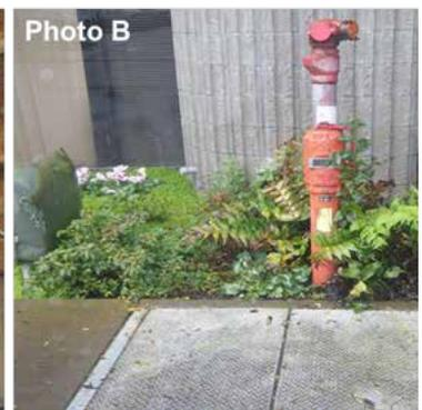
Photo A shows the typical piping of a commercial building sprinkler system near the roof line of the building. Photo B shows the protection system valve, which is commonly found at the exterior of a building with a fire suppression system installed.
