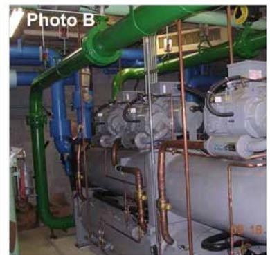
The photos above show the variance in the size of chiller compressors in commercial buildings. Photo A is the compressor of a smaller, older style of chiller. Also notice the oil leaking from the older compressor in Photo A. Photo B is the compressor for a newer, much larger chiller.
