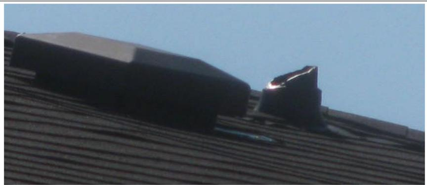
*This vent stack does not go through the roof far enough, so it could freeze over or become full of snow.*
