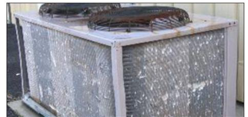
Sometimes the inspector discovers air-conditioning units that are badly damaged by hail. On one warehouse inspection, an inspector found that all of the rooftop air-conditioning units were damaged by hail or were missing altogether, possibly due to theft.
